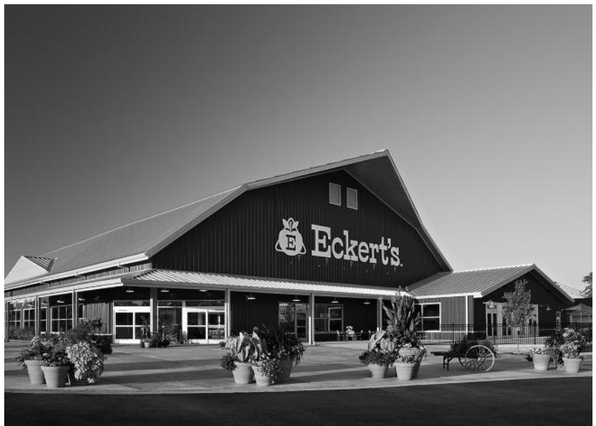
▲ The newly expanded Eckert's in Belleville, where additional investment is being made by IDOT in a new entrance.
